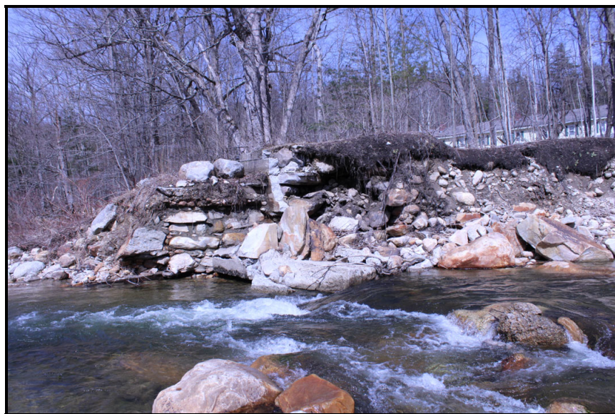
Figure 9. A short portion of an older dam has been exposed by erosion of the right bank.
