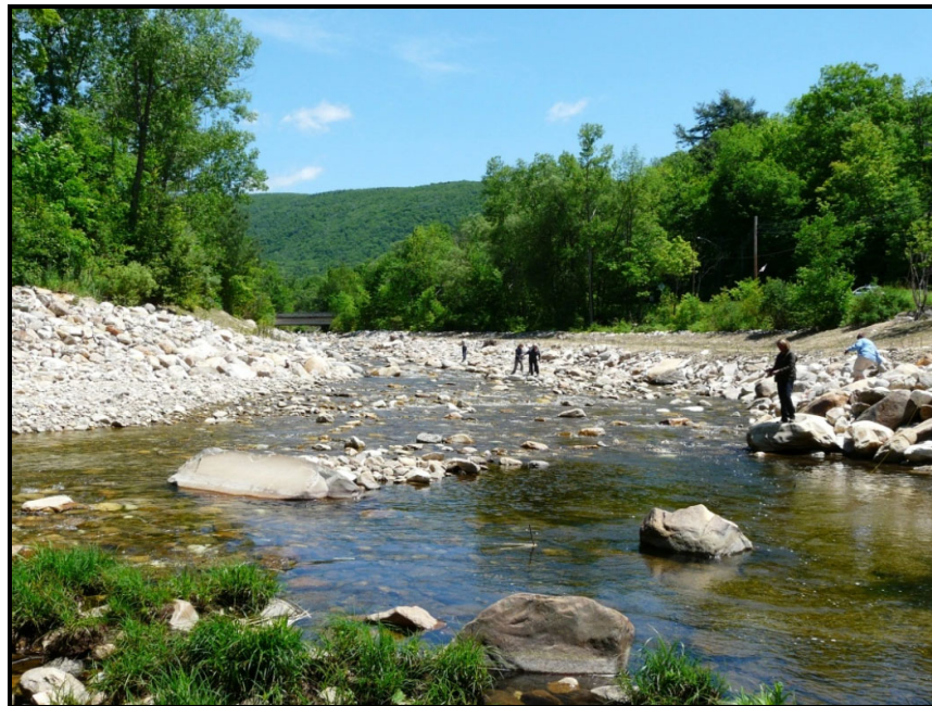
Figure 5. Looking upstream through the old dam site at the excavated channel and inset floodplain constructed upstream of the former dam prior to Tropical Storm Irene. (From Web citation 3)
