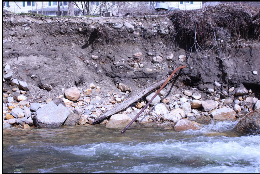
Figure 8. The eroding right bank upstream of the former dam is composed of artificial fill.
