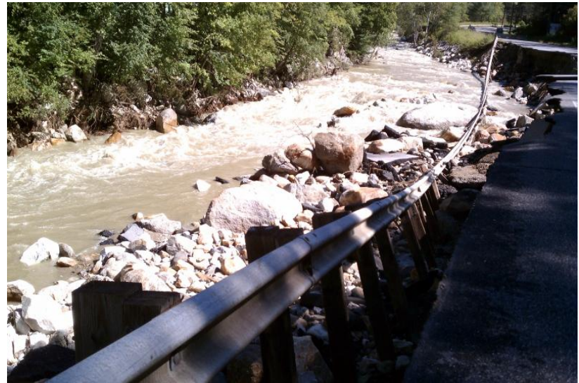
Fig. 3.5. Damage to River Road (Rt. 8) from T.S. Irene
