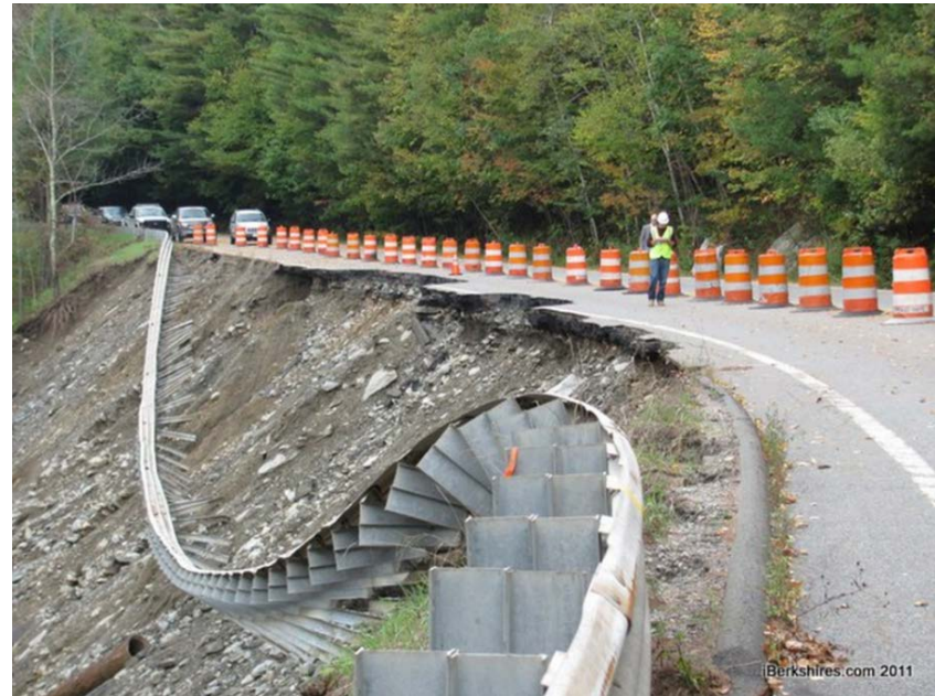
Figure 3.19. Mohawk Trail (Rt. 2) damage from T.S. Irene
