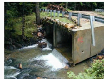
Bridge in Worthington had history of falling. In 2003 road washed out and was closed to all traffic.
