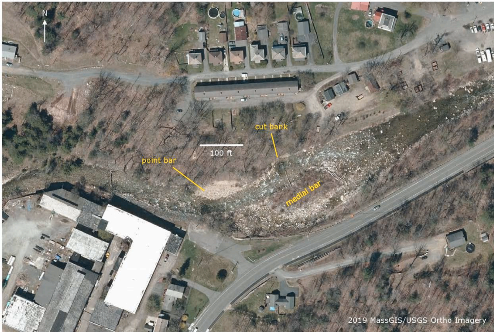
Fig. 3.11. North Branch Hoosic River showing lateral movement in proximity of Carson Avenue structures
