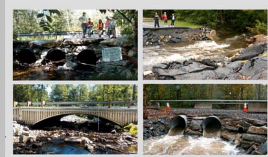
Clockwise from top left: First replacement crossing (2009); catastrophic culvert failure due to Tropical Storm Irene (2011); "emergency temporary replacement" crossing (2011); replacement bridge (2016).
