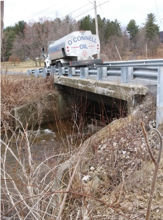
Figs. 3.6-3.7. Cross Road Bridge has deteriorated to the point that it is down to a one-lane road.
