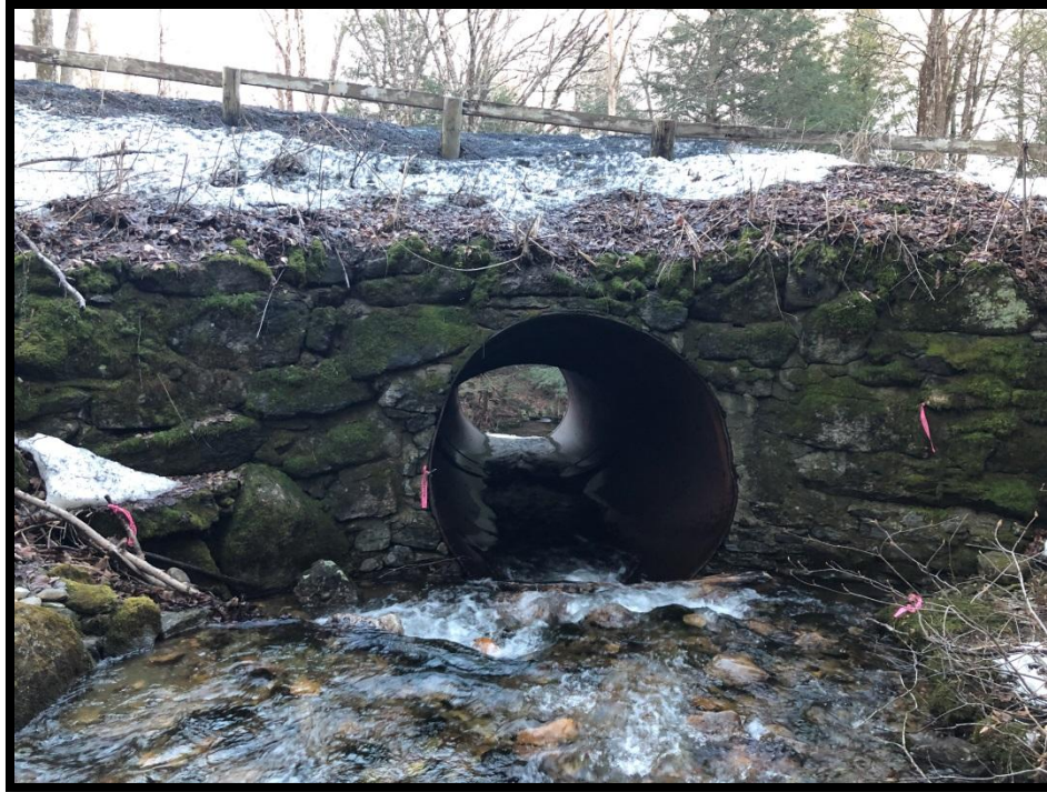
Photo 2: Displays the existing headwall and culvert inlet under West Road from an upstream perspective.
