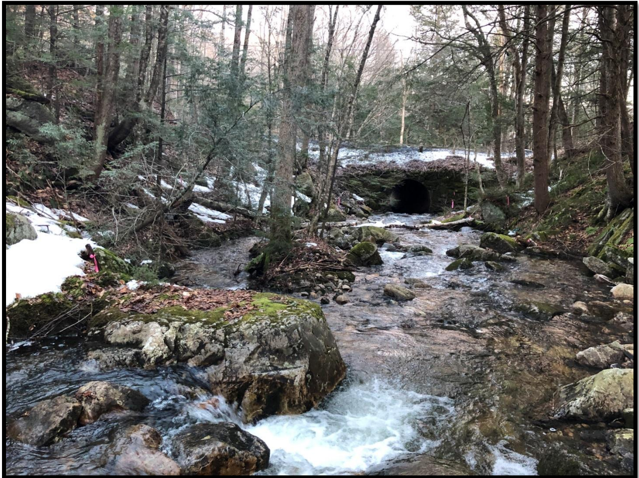
Photo 1: Displays Bear Swamp Brook and the existing culvert under West Road from an upstream perspective.
